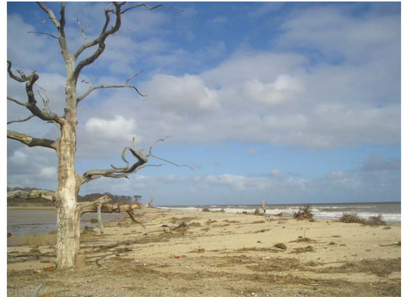
Imminent permanent breaching of beach barrier, Covehithe, Suffolk, 2007.
